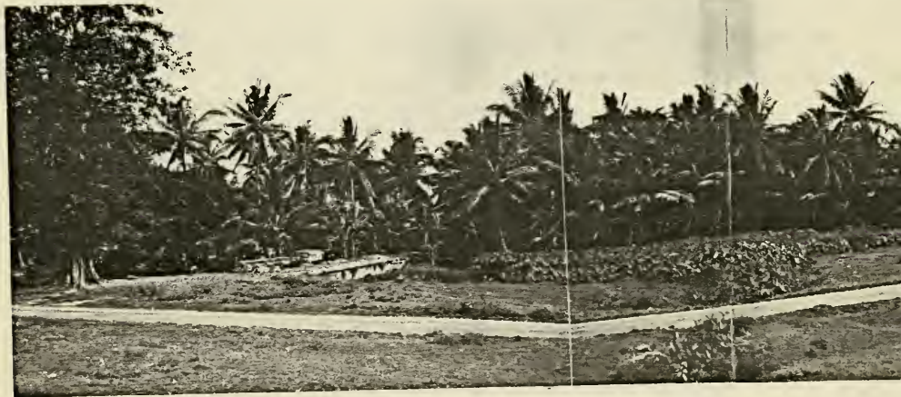
The southern part of Surosowan fortress which shows the canal and the old bridge connecting between Surosowan Palace and Tasikardi. Photographed by Dina Darmawanti, 1985
